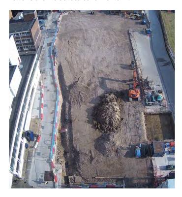
During the excavation works an unplotted water main was found in the South West corner of the site which clashes with the new foundations. We will be diverting this main without any interruption to the supply of the surrounding buildings.
