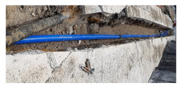
A new trench was excavated outside our future working area, in which a new 4" MDPE pipe was laid. Before the existing pipe was disconnected, a 2" bypass pipe was installed that ensured the flow of water was maintained whilst the diversion took place.
