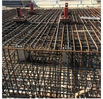
The crane base works are on target for the crane delivery on the weekends of 4 and 11 July 2020. There is a considerable amount of rebar, which form a cage to reinforce the concrete and allow the cast-in crane anchor that the cranes are connected with, to be tied down when they arrive on site.
