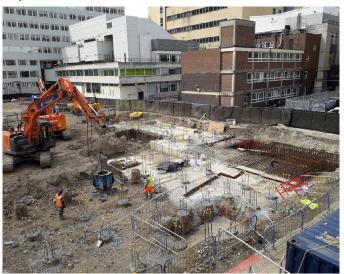
The crane bases are both now poured and cured, and tower crane 1 will be erected over this forthcoming weekend, subject to wind conditions. The fully erected crane will then be roped up and tested, and will be operable from early next week.
