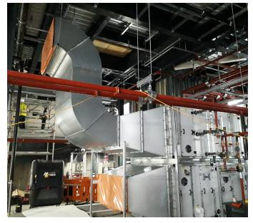
On the eighth floor level, some large plant items such as the boilers and AHUs have been fitted, and the high level pipework, ductwork and mechanical services are currently being installed. Cable tray hangers are fixed, ready for the large cables to be pulled up from the LV switchroom at ground level.
